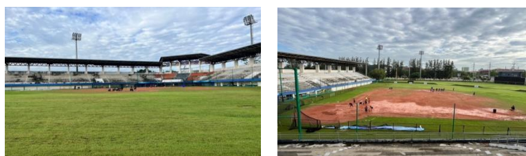
Baseball – Softball Stadium, Queen Sirikit Sports Center
